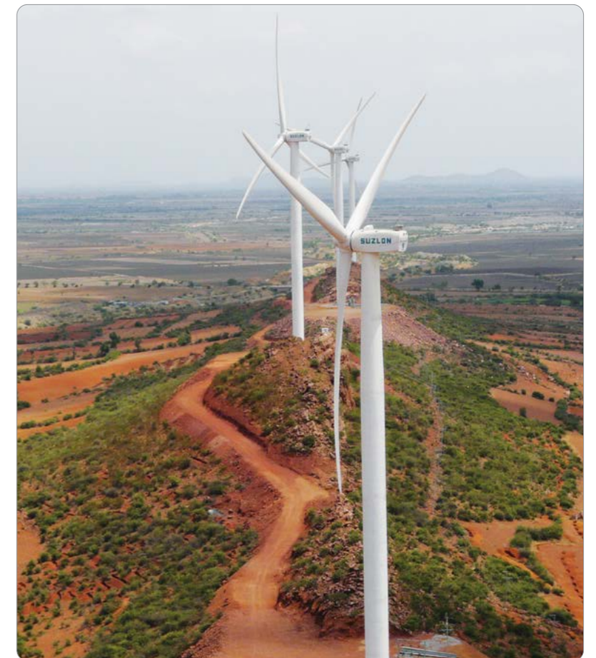
A Wind Power Plant in Andhra Pradesh
