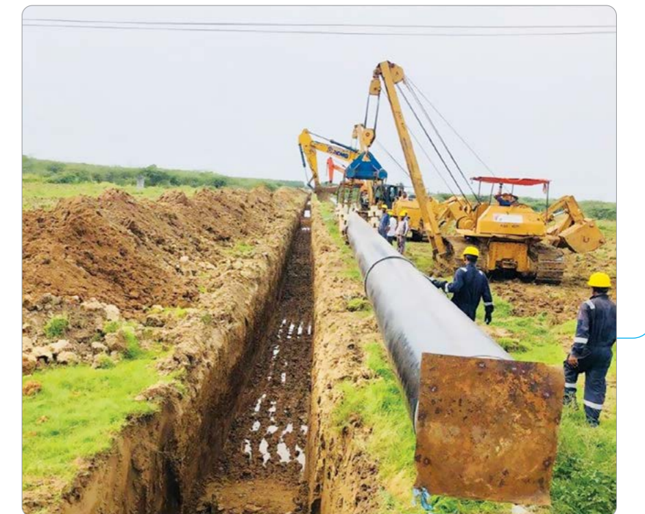
Underground Pipeline being laid in southern part of India
