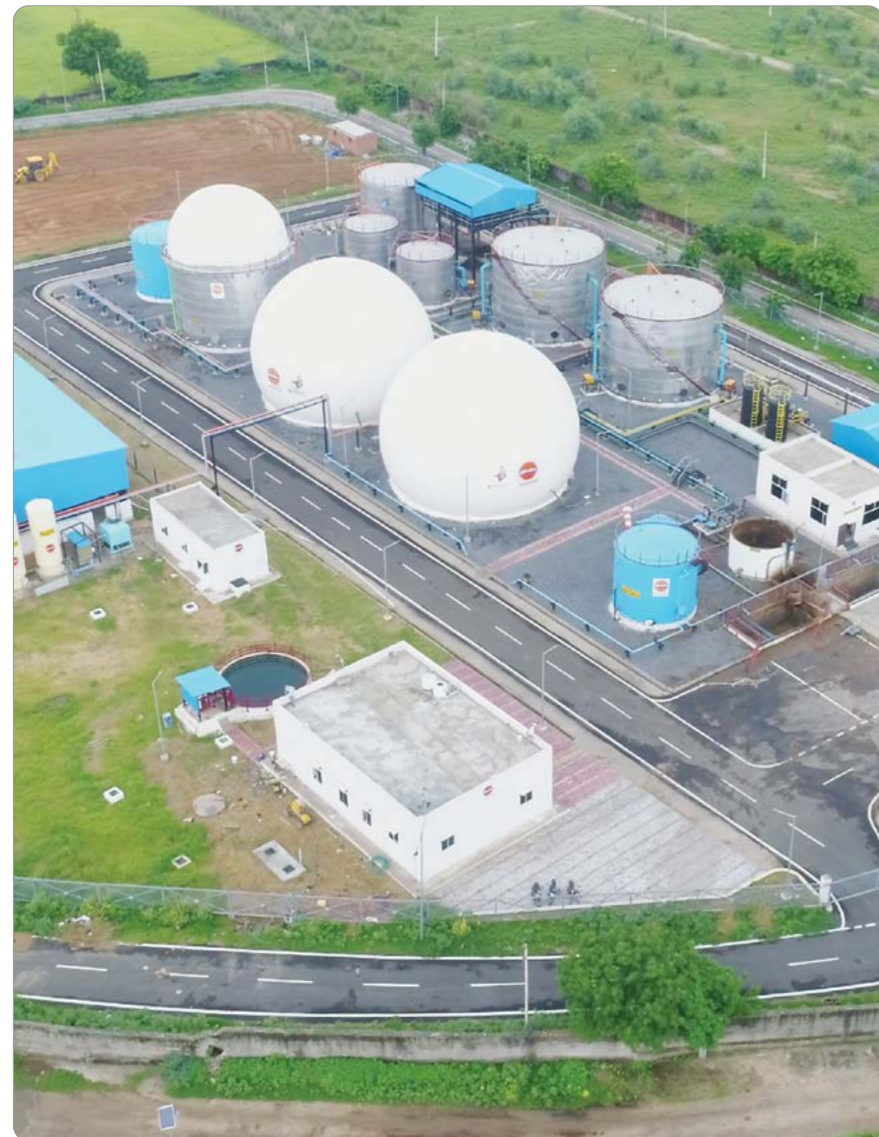
Compressed Biogas plant at Hingonia, Jaipur
